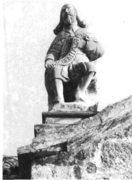
Kip proroka Jeremije na zabatu sjevernog pročelja Statue of the prophet Jeremiah on the gable of the northern facade
