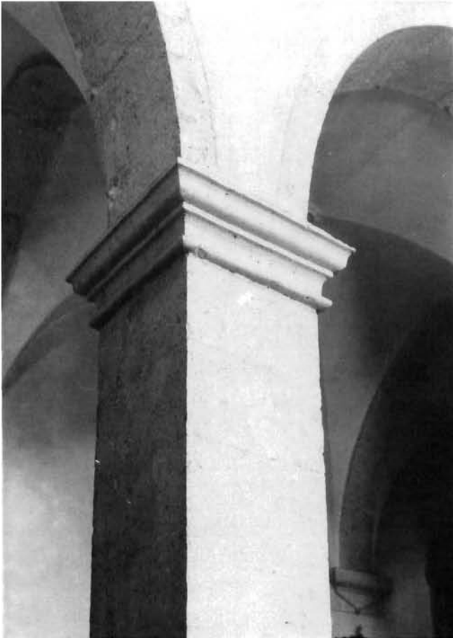
Nosač arkada s pojasnicama i svodovima broda Arcade abutment with arch bents and nave vaults
