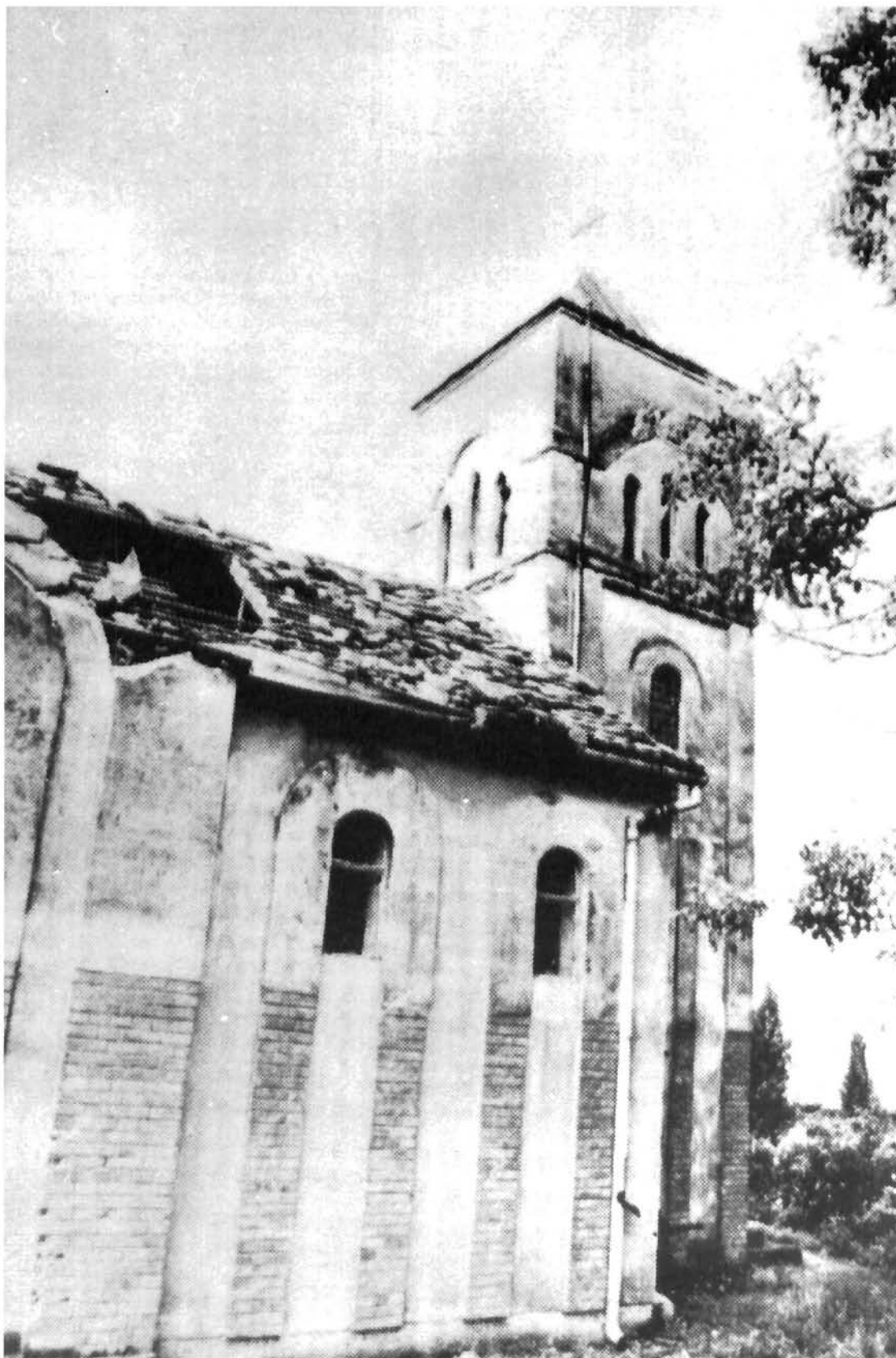
Erdut, pravoslavna crkva pogodena granatom JA, srpanj 1991. (foto: Jozo Petrić) Erdut, the Orthodox Church hit by Yugoslav Army shells, July 1991. (photo: Jozo Petrić)
