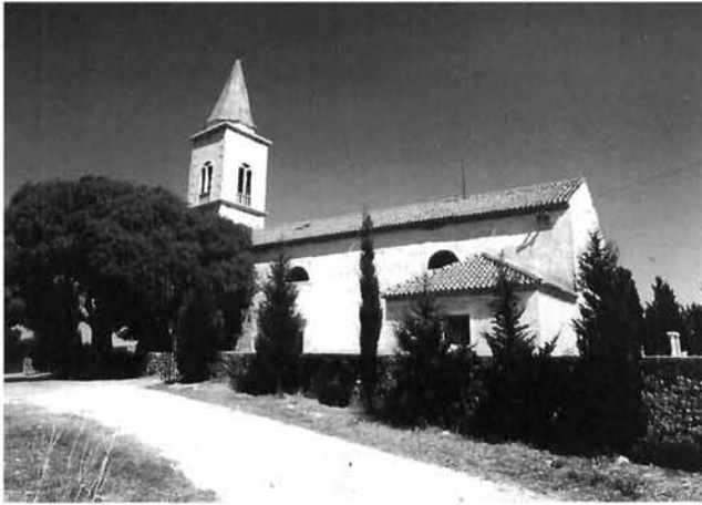
Crkva Uznesenja Blažene Djevice u Ugljanu, početak 18. st.; pogled na južno lice i sakristiju. Zvonik podignut oko 1976. g. Church of Our Lady's Assumption in Ugljan, beg. 18th c; view of south front and sacristy. Front steeple built in about 1976
