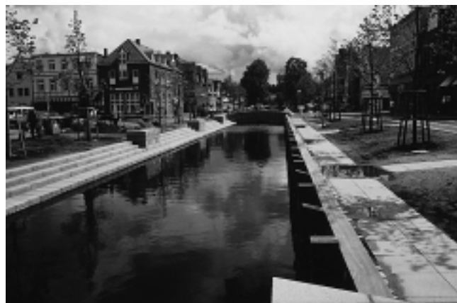
Glückstadt, »Am Fleth« s uredenim kanalom Glückstadt, "Am Fleth" after the canal was reinstated.
