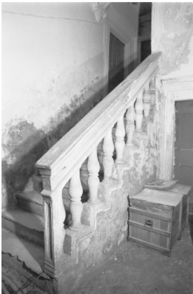
Predvorje, balustrada stubišta Entrance hall, staircase balustrade
