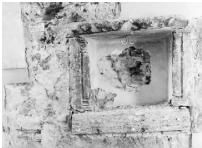
Pilo u kuhinji četvrtog kata Fourth-floor kitchen sink
