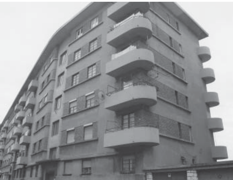
Stambene zgrade u Laginjinoj ulici 31 i Tizianovoj ulici 1 i 3, pročelja Residential buildings in 31 Laginjina street and 1, 3 Tiziano street, façades
