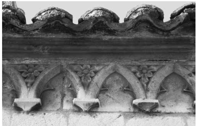
18 Slijepi lukovi potkrovnih vijenaca kapelica Blind arches under the cornices of the chapels
