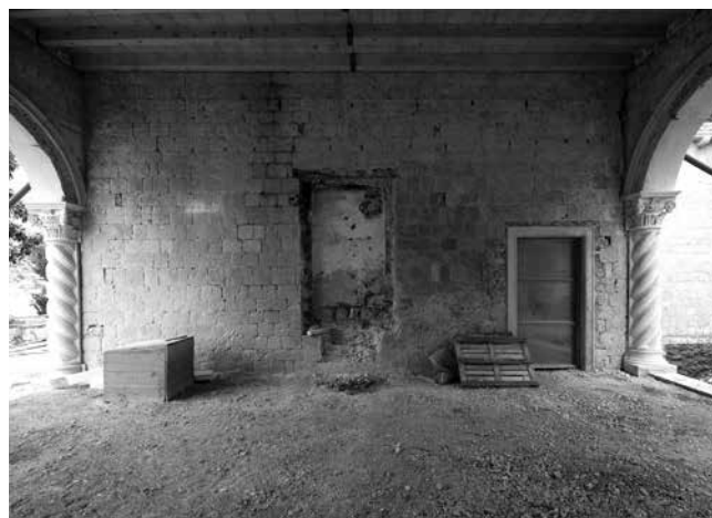
13 Nalaz zidnog umivaonika u istočnom zidu lođe (foto: N. Vasić, Hrvatski restauratorski zavod) Remains of an in-built washing basin in the eastern wall of the loggia (photo: N. Vasić, Croatian Conservation Institute)
